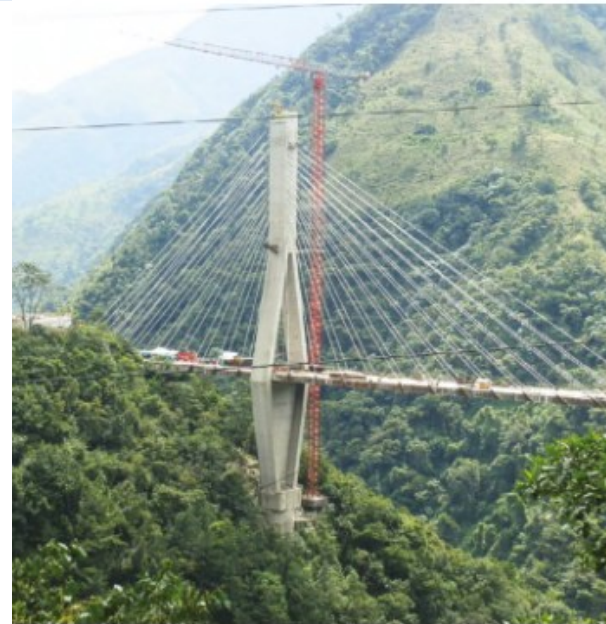
Pylon C, identical to Pylon B, of the cable-stayed Chirajara Bridge
