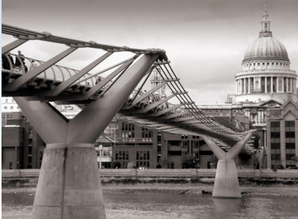
Millenium bridge, 2000, London, UK
