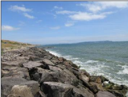
Rock armour revetment
